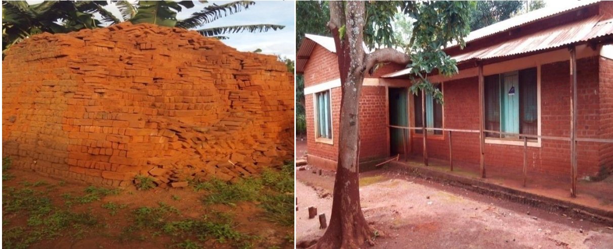
Photo 2: Use of burnt bricks in building construction (Photo by Lukando, April 2015).
