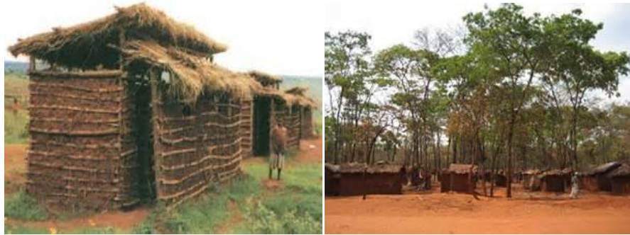
Photo 1: Use of poles and thatch grass in construction of temporary houses for refugees (Photo by Lukando, April 2015).
